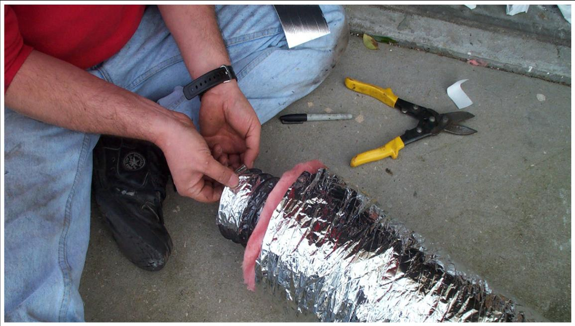
After trimming to proper length, take the newly exposed end, and reinforce it just like the other end. It would be a shame to lose cold air in the insulation should your ducting tear.
