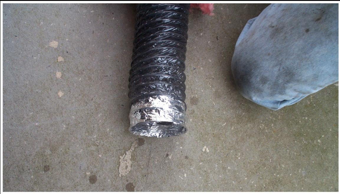
**First, roll or push the insulation back to reveal the ducting itself. The end should appear fairly fragile, so we reinforced it with mylar duct tape. Use whatever you have to make the end sturdy. As the inlet, you want it to be able to handle whatever speed air is thrown up through your intake.**
