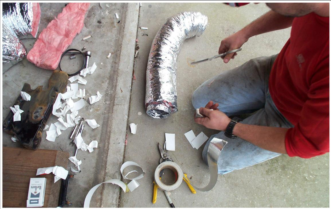
Here we have Carl and mylar tape again. He's cutting off pieces to secure the insulation and outer layer to the inner.
