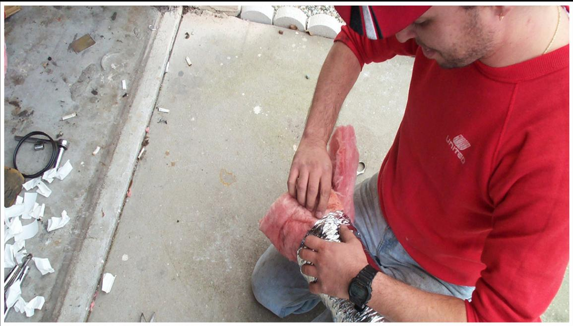
When you've gotten to the end, you'll doubtlessly have "leftover" insulation at the end. Simply cut and remove this extraneous material, and consider yourself almost finished.
